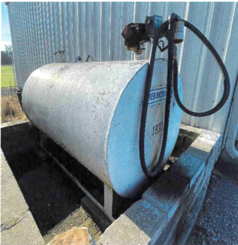
Figure 10: 500-gallon diesel AST
